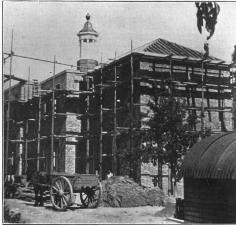
THE NEW LAB. BLOCK.
